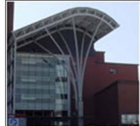
Toronto Western Hospital
