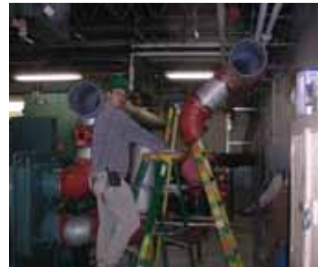
Chiller pipe being installed at the Queensway-Carleton Hospital.
