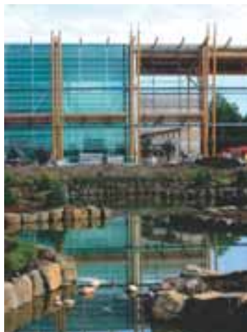
Storm water management and the gardens at the Café at the new Thunder Bay Regional Health Sciences Centre.
